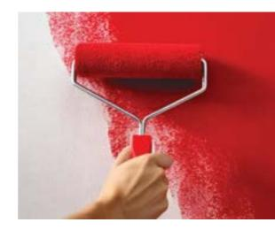
Once the surface is smooth and solid, apply NESCOAT® PUREPRIME transparent primer on absorbent surfaces such as gypsum plaster, and NESCOAT® INPRIME interior wall primer on all other surfaces in a single coat. After the primer application, the surface should be allowed to dry for at least 12 hours before proceeding with the paint application.
