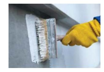
The product gains mechanical strength 3 days after application and becomes waterproof 7 days after application. Curing time shortens at higher temperatures and lengthens at lower temperatures.
