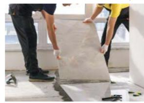
Gradually add 25 kg of NESCOAT® SUPERFIX FLEX to 7-7.5 liters of clean water and mix with a low-speed mixer for approximately 3 minutes until a lump-free consistency is achieved. Let the mortar stand for 5 minutes to allow the additives to dissolve, then mix again for 1 minute. If necessary, adjust the consistency by adding a small amount of water or product. The prepared mortar should be used within 4 hours. Do not add water or product to the hardened material.
