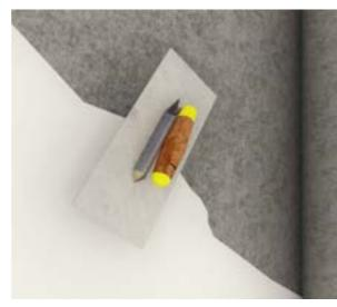
The substrate must be clean, dry, and structurally sound to support the application. In restoration works, weak plaster layers should be mechanically removed entirely. Cracks should be widened in a V-shape to reach stable areas. The surface should be cleaned of dirt, dust, and other adhesion-impairing materials. The surface should be dampened without allowing water pooling. Highly absorbent surfaces should be primed with NESCOAT® **PUREPRIME** transparent primer before application.
