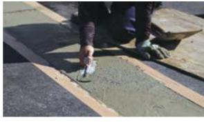
MORTAR PREPARATION Gradually add 25 kg of NESCOAT® GROUT PLUS into 3.5-4 liters of clean water (14-16% water by weight) while mixing with a low-speed mixer. Mix for approximately 3 minutes until a lump-free consistency is achieved. Use the prepared mortar within 30 minutes, and only prepare the amount that can be used within this time frame. Do not add water or product to reuse hardened material.
