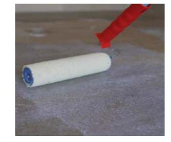
**NESCOAT® UNIRIME**, is ready to use and should only be stirred until a homogeneous consistency is achieved. The product is applied in a single coat using a roller or brush. After the primer application, wait at least 12 hours for the surface to dry before proceeding with the coating process. After application, hands and tools should be thoroughly cleaned with plenty of water. **DRYING TIME** • Surface drying: 6 hours at 23 °C and 50% relative humidity. • Full drying time: 24 hours.
